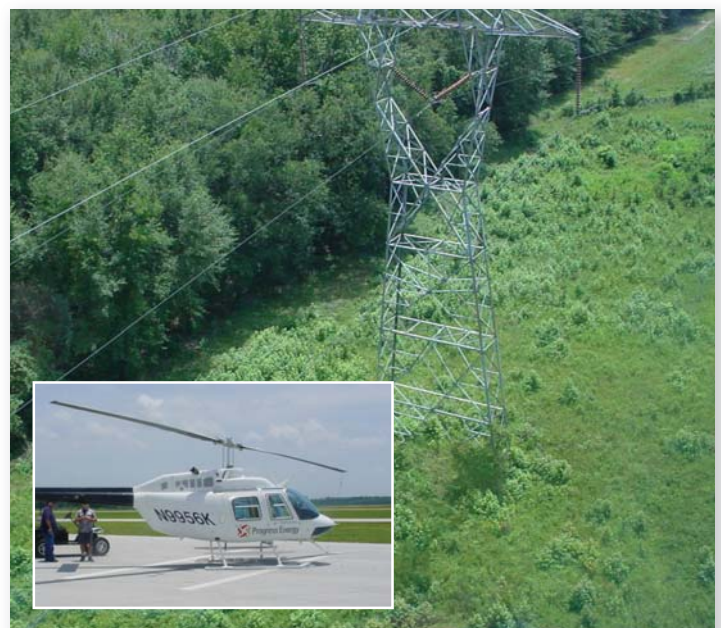
Aerial patrols are the quickest way to inspect transmission line ROW. Progress Energy does most of its aerial inspections with a helicopter.
