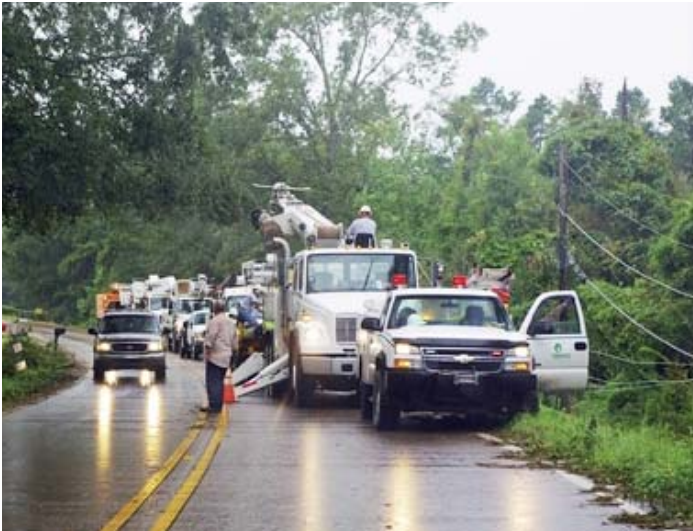
Crews work to restore power after a major storm.
